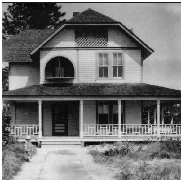
Reed House (1925) Oleander Avenue, White City
